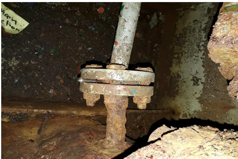
Corroded shaft cooling line
