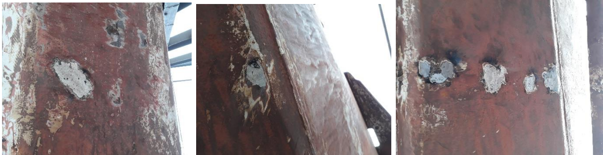
Cavitation filling
